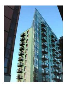
Owing to variable positioning of the mullions which altered with the height and width of the prow, continuous vertical drainage could not be achieved between floor levels. Acoustic separation also required some form of physical break in the system at each apartment level. Both of these performance parameters were addressed by means of Schuco split transoms.
